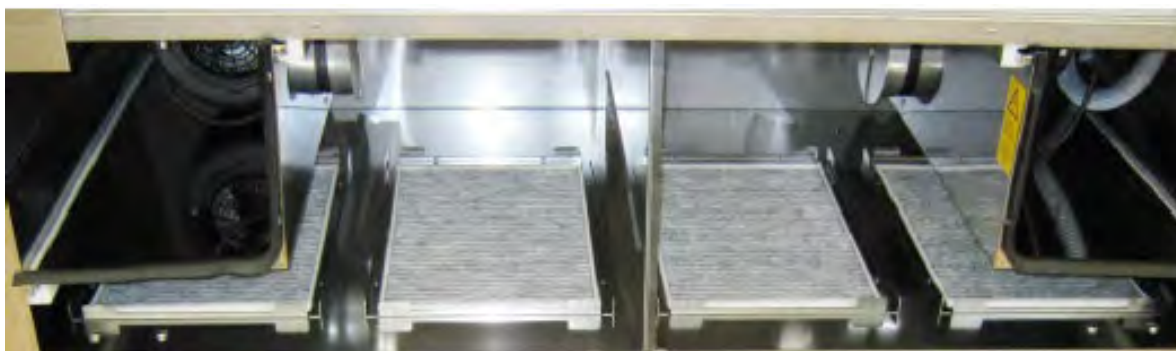
Arrangement of the activated carbon filters (number depending on model)
